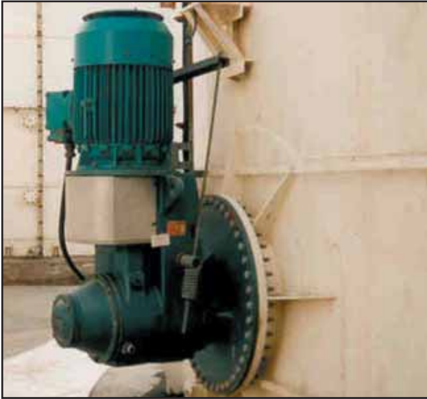
Fixed Angle Mixers Installed in a refinery for a blending application.
