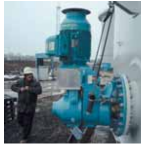
Swivel angle gear driven mixer installed in a Russian refinery.
